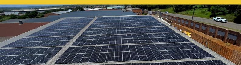
**Storage Facility, Johannesburg:** 115kw capacity is powered by a combination of 144 panels, 3x50kW Deye Inverters, and a 120kWH Deye HV battery. This innovative grid-tied system allows for both energy consumption and storage, offering resilience against power outages and potentially generating income by selling excess energy back to the grid.
